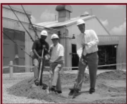
DuPont Ground Breaking Ceremony
