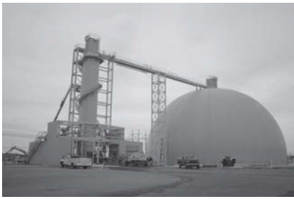
Product Storage Dome at the Northeast Carbon Burn-Out Facility.
