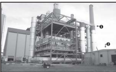
Month 9 - Ductwork installed, electrical and control system installation continue.
