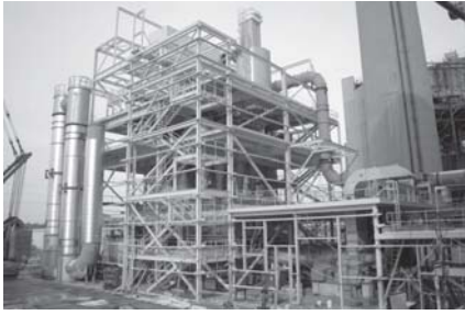
CBO Tower at the Northeast Carbon Burn-Out Facility.
