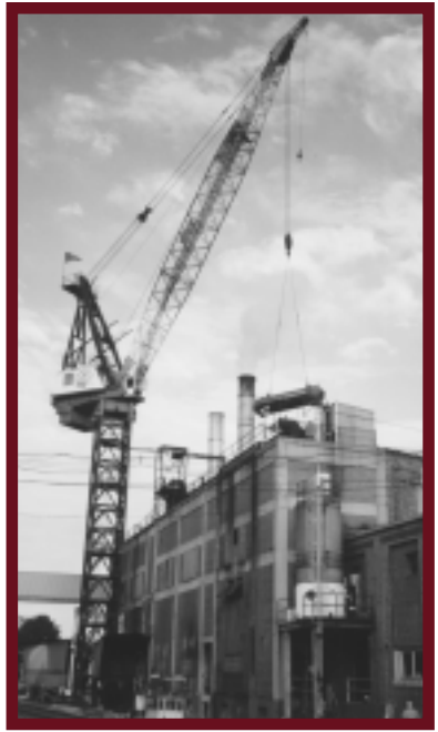
Figure 2. Setting of the 48,000 pound steam drum utilizing an 86-ton tower/gantry crane.
