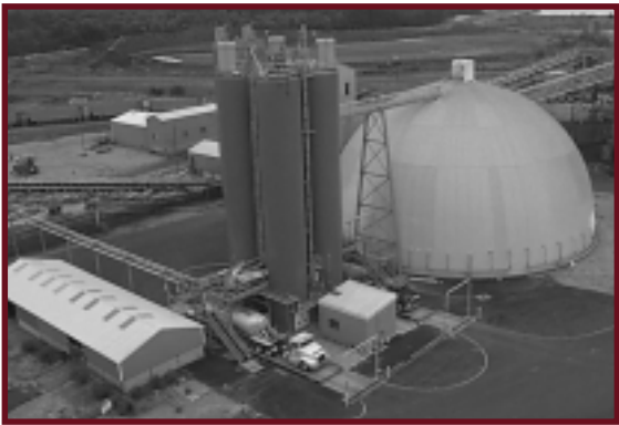
The storage loadout area consisting of the loadout silos and the storage dome.
